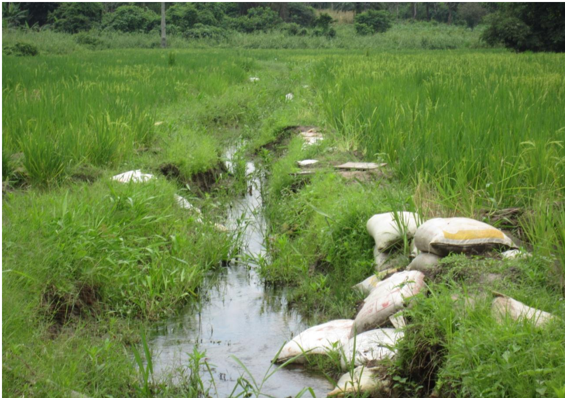
Plate 10: Leakages here and there 8 weeks after repairs of central drainage canal
