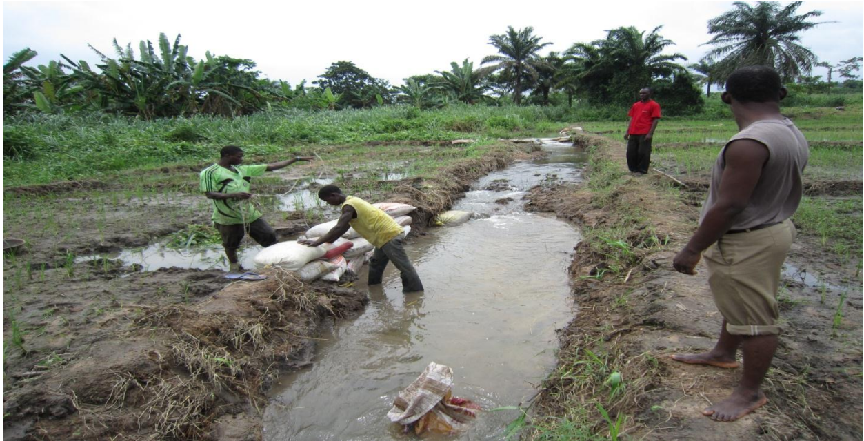
Plate 9: Commencement of repairs
