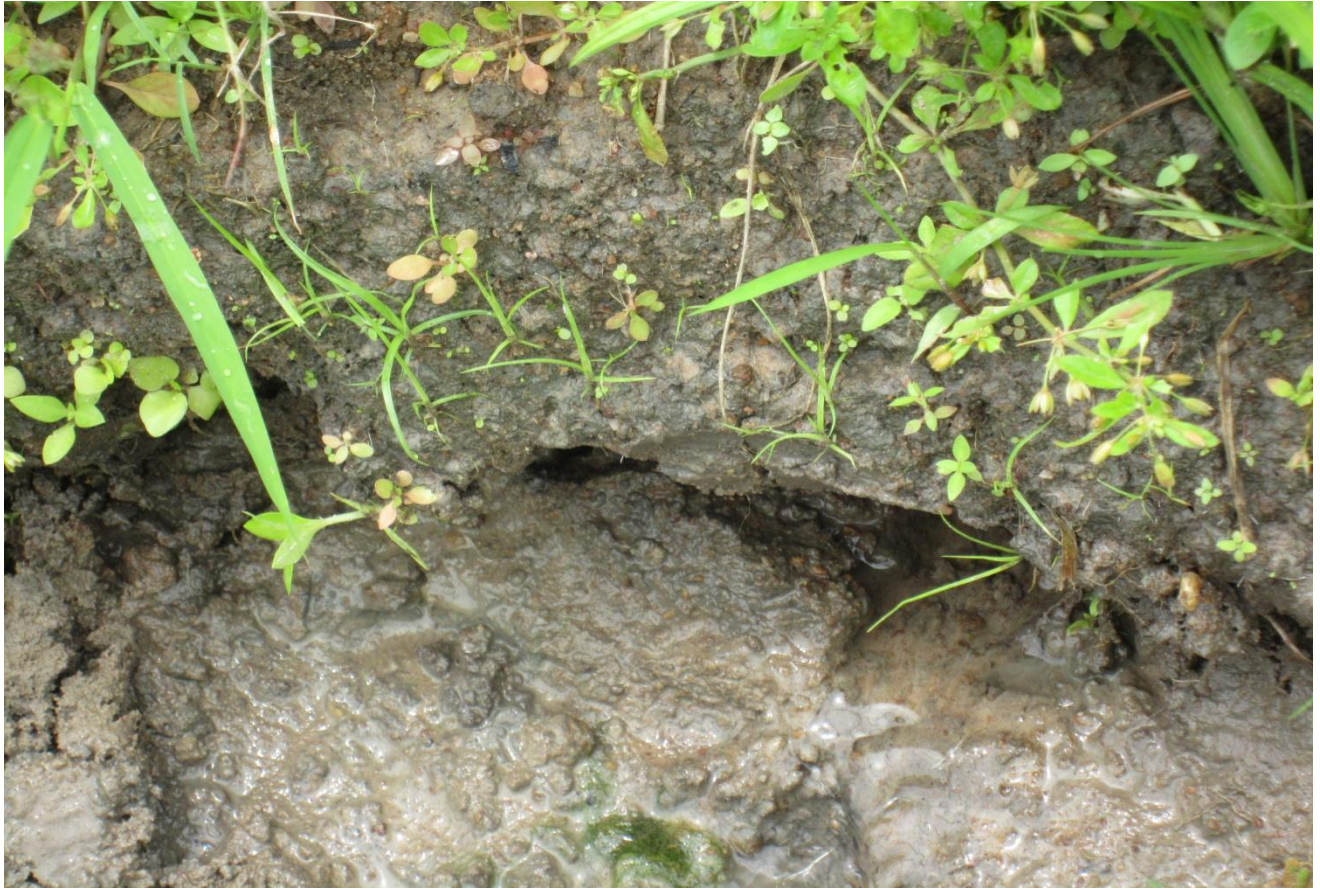
Plate 11: Weakened bunds with leakages after repairs
