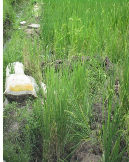
Plate 13: When bund repair with sand bags and soil failed, another bund inside each sawah unit was done but leakages persist.
