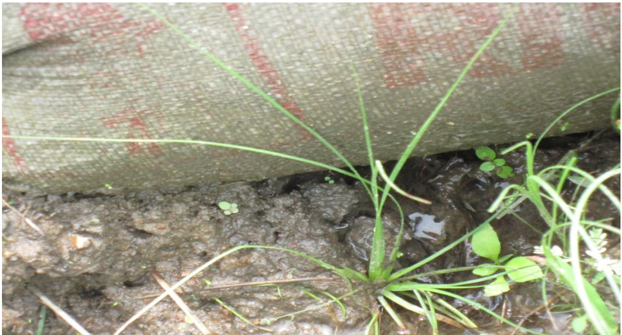
Plate 12: Leakages in the mended bunds
